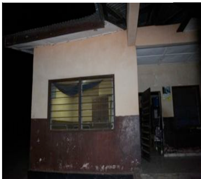
Newly lit maternity ward at Bamoi PHU during night
