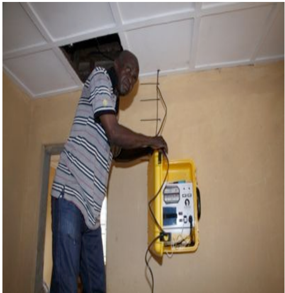
Technician installing the solar suitcase in Bamoi PHU
