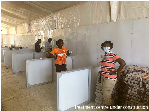
Treatment centre under construction
